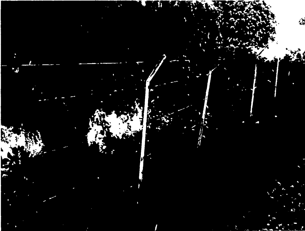
Solar Fencing in Athmallik Division
