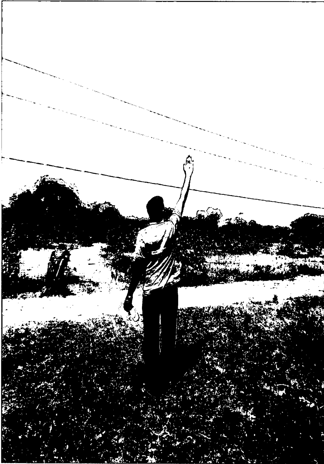
Sagging of electric line, Dhenkanal Division
