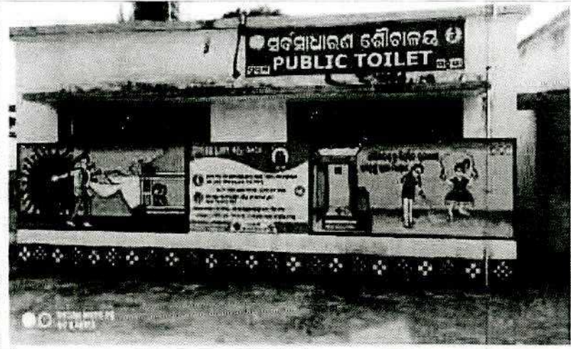
Toilet Block at CHC, Beltikri
