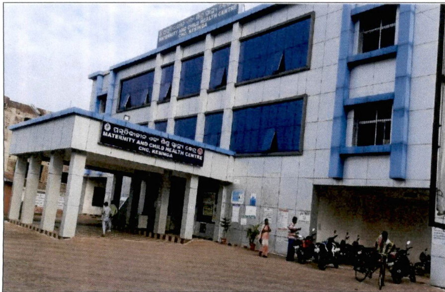
MCH building CHC Kesinga
